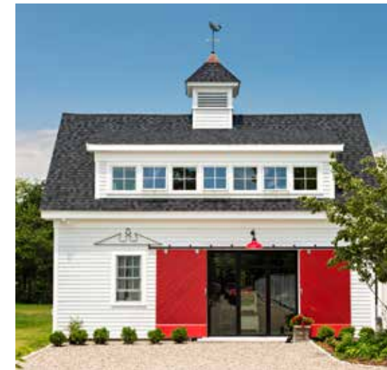
THE BARN DOORS, painted a cheery red, roll open to reveal a NanaWall glass door system (LEFT). The new shed dormer has a series of divided awning windows that seem architecturally appropriate for the old building and allow lots of natural light into the second-floor office space (ABOVE LEFT). On the lower level, simple wood shelves by the stairway (ABOVE RIGHT) pick up on the rustic vibe.
